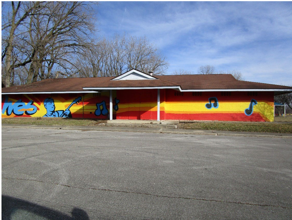
View looking east at community center
