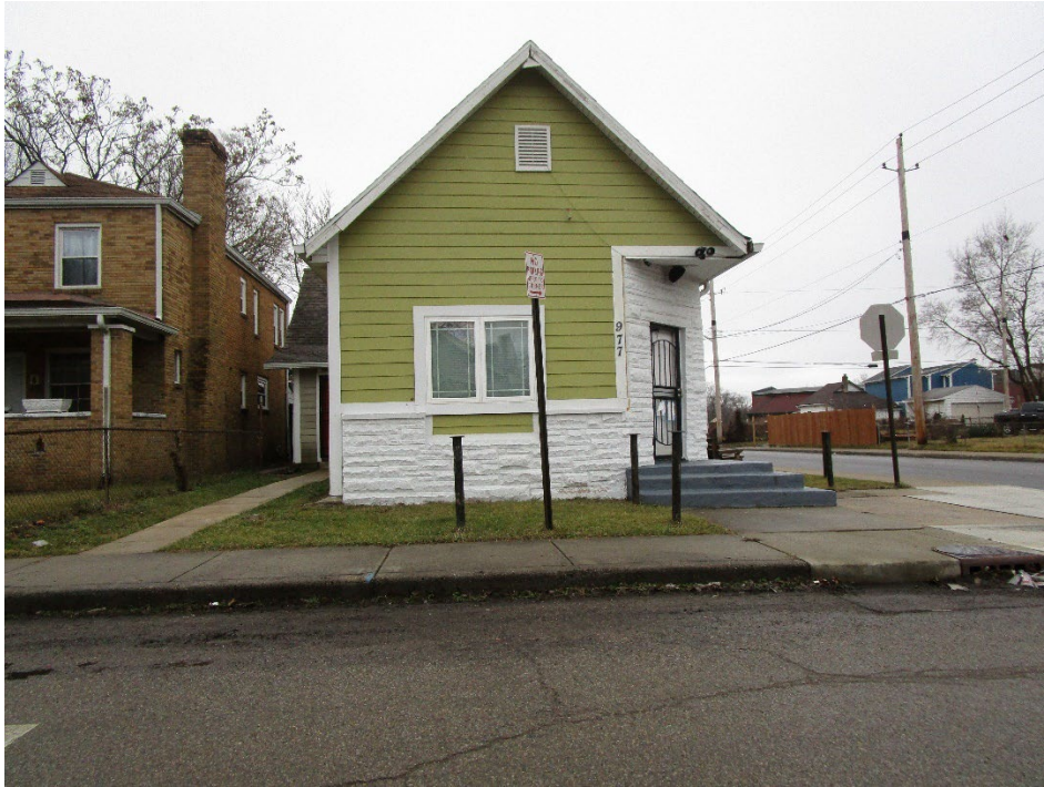
View of site looking south across Roache Street
