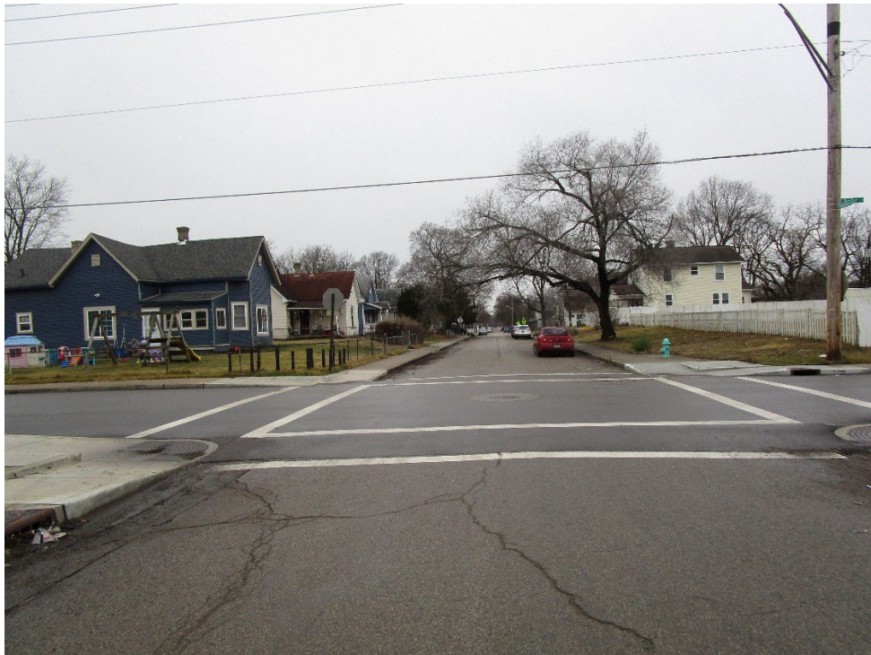
View looking west along Roache Street
