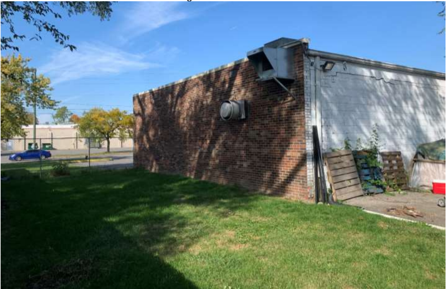
Photo of the existing southern building façade.
