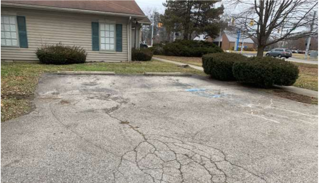
Two parking spots on site that would need to be restriped.
