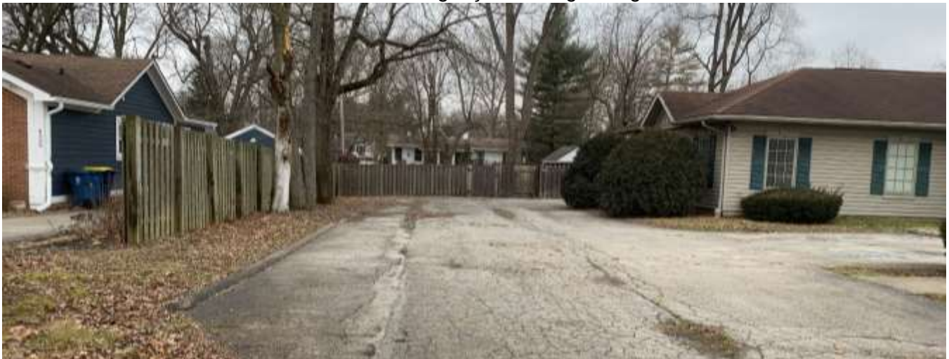
Photo of the existing parking lot on site.
