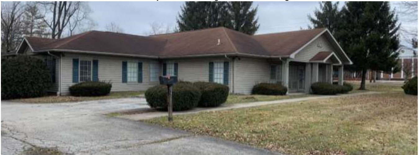
Photo of the front building façade facing College Avenue.
