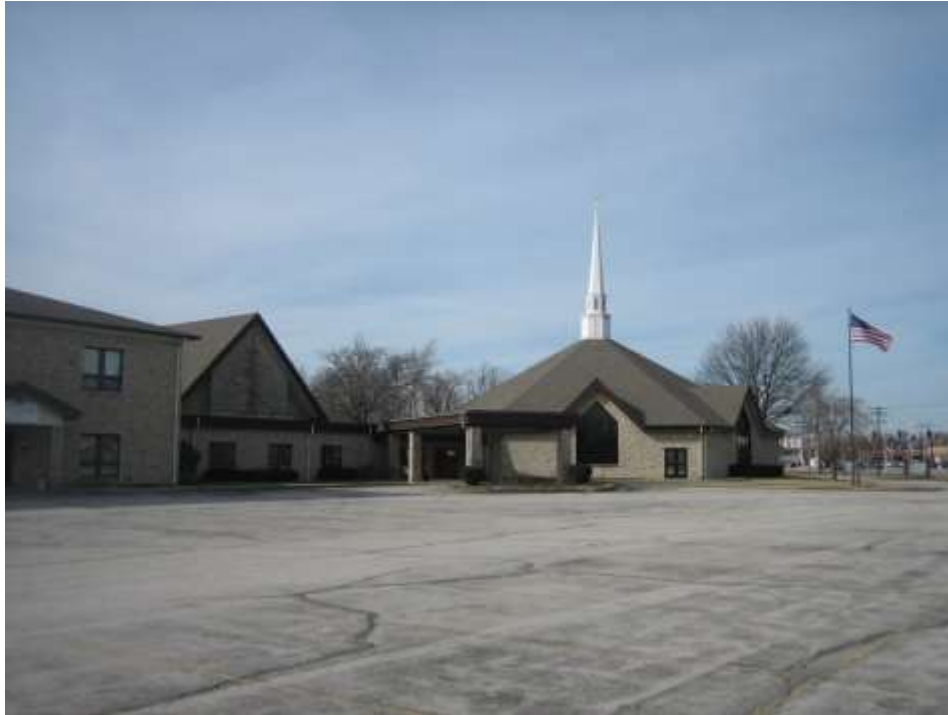
Subject site building, looking north
