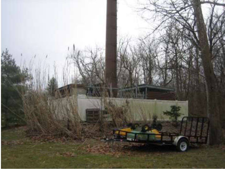
Existing wireless communication facility with 2.5-foot west rear setback, looking east
