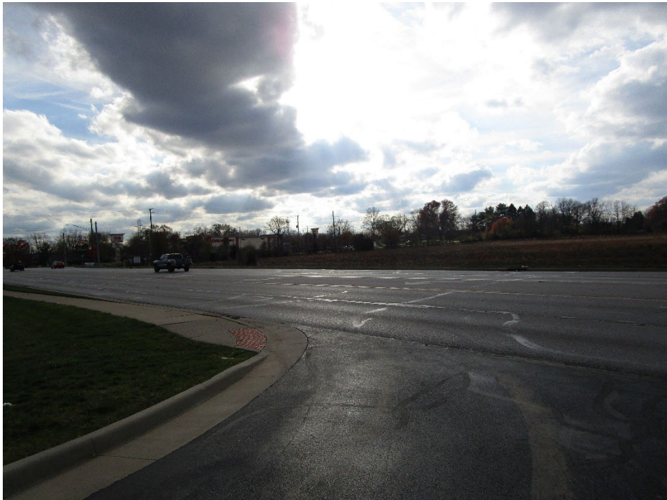
View of site looking southwest across South Emerson Avenue
