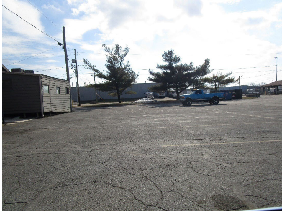
View of site looking south
