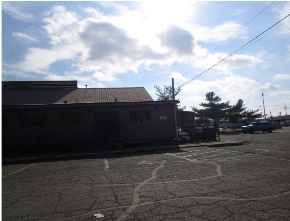
View of site looking south
