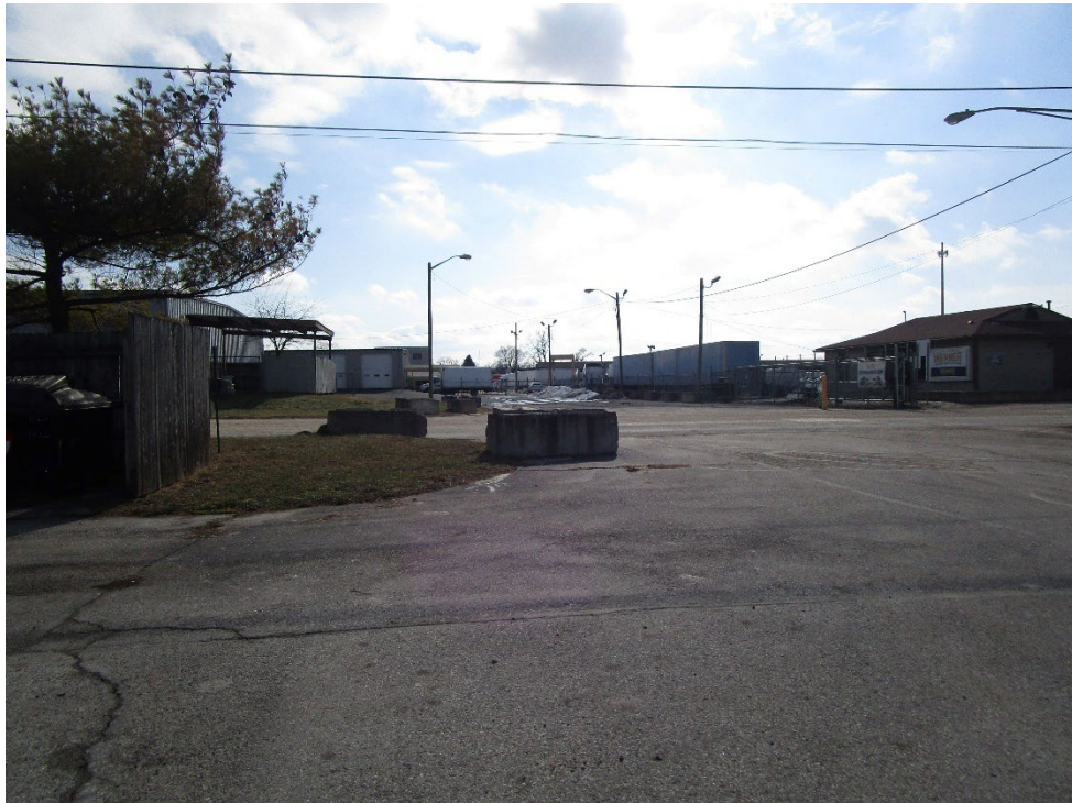
View from site looking south
