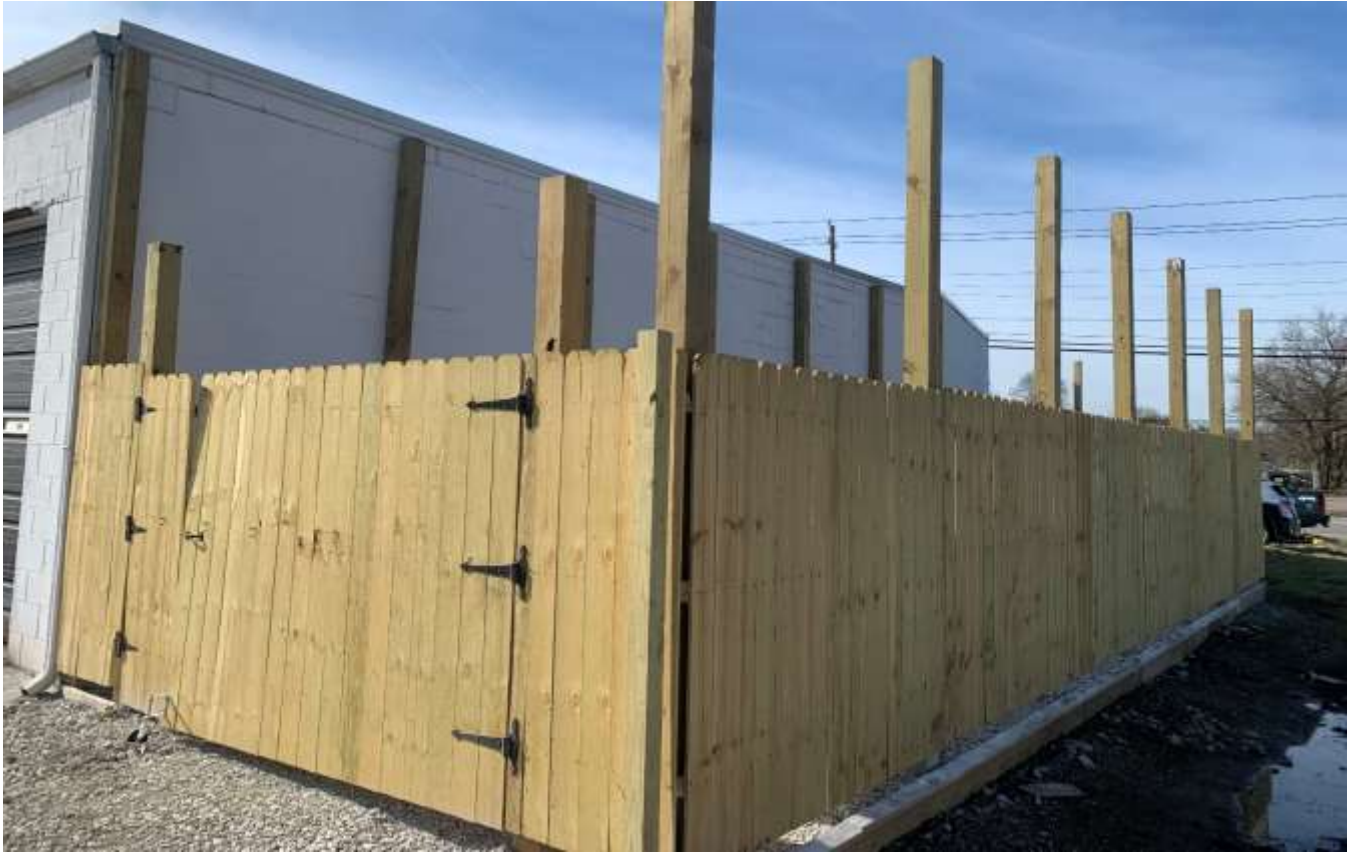
Photo of the removed building addition on the north side of the building.
