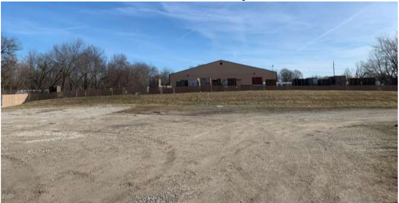
Photo of the property east of the site.
