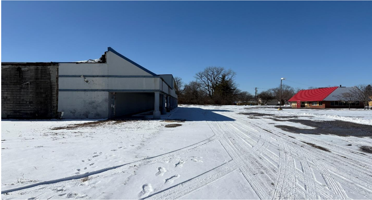
Photo Eleven: Looking West, Southernmost Structure to the Left
