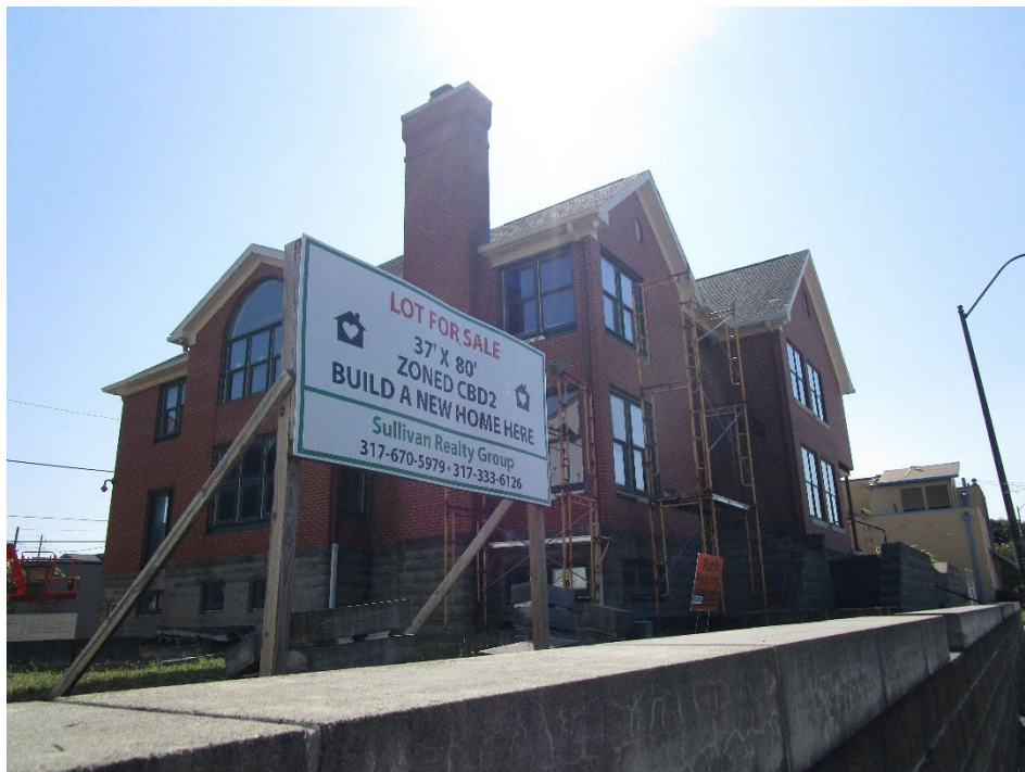
View looking southeast at adjacent two-family dwelling
