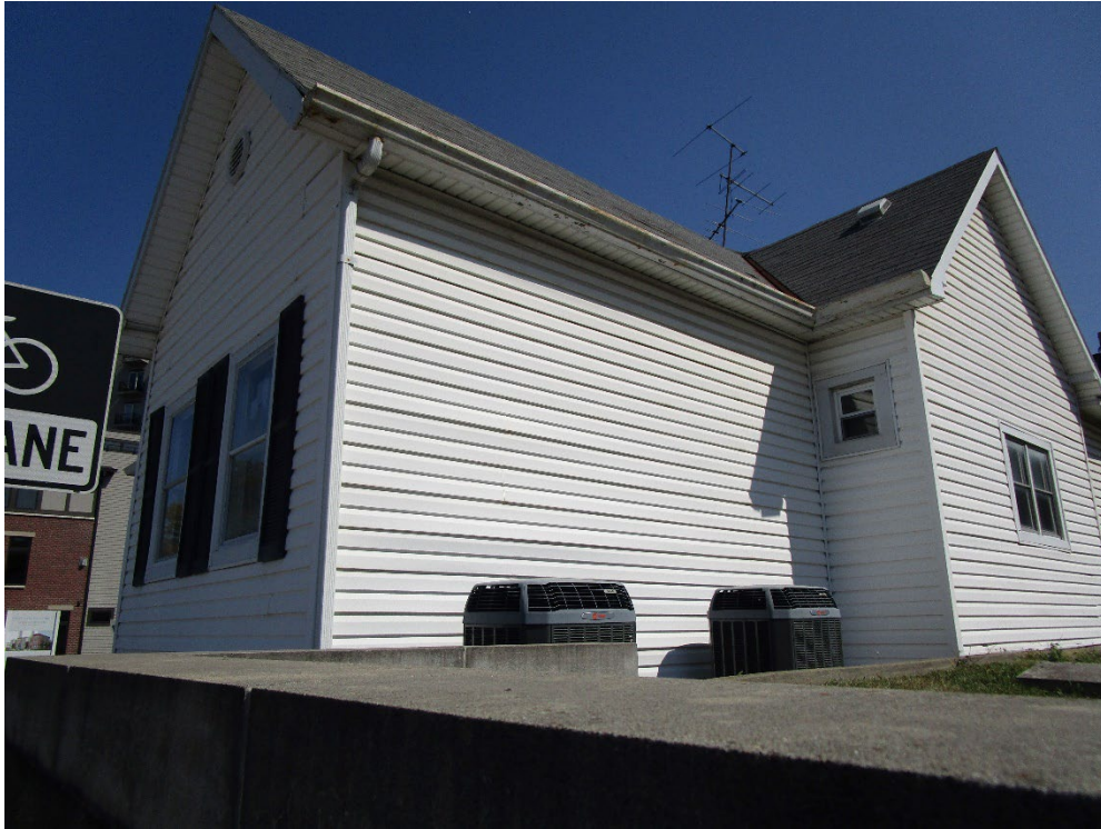
View looking northeast at adjacent single-family dwelling
