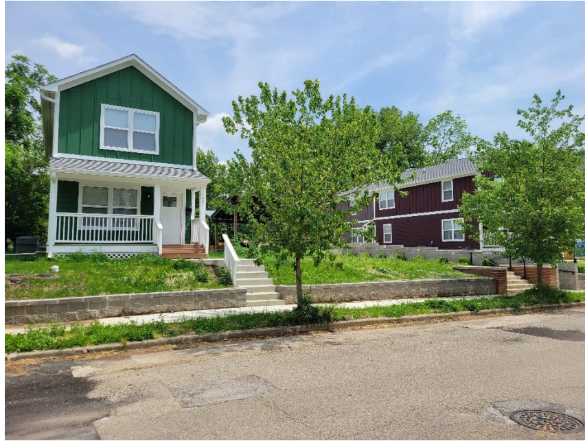
Photo 5: Both Structures Viewed from West
