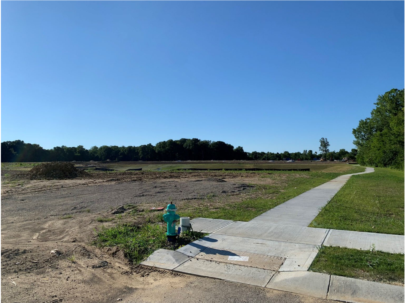
Photo of Section 3A from Elden Drive, looking northwest
