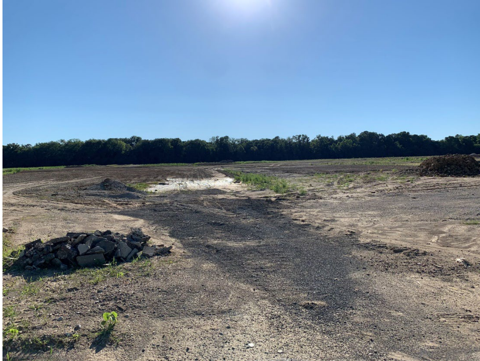
Photos of Section 3A, from Elden Drive, looking west
