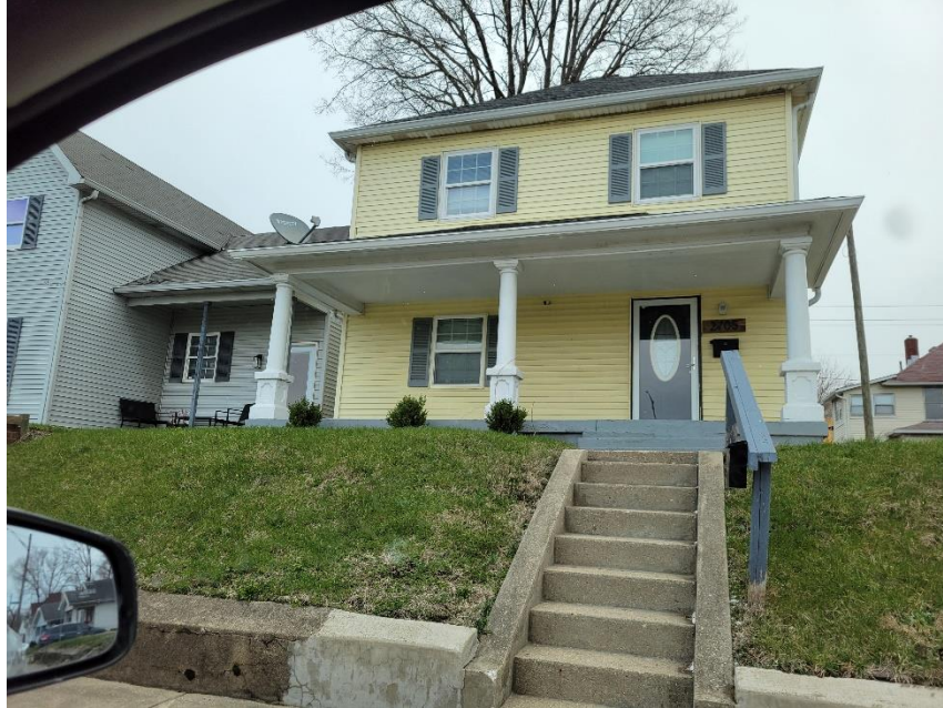
Photo 1: Subject Site Viewed from West
