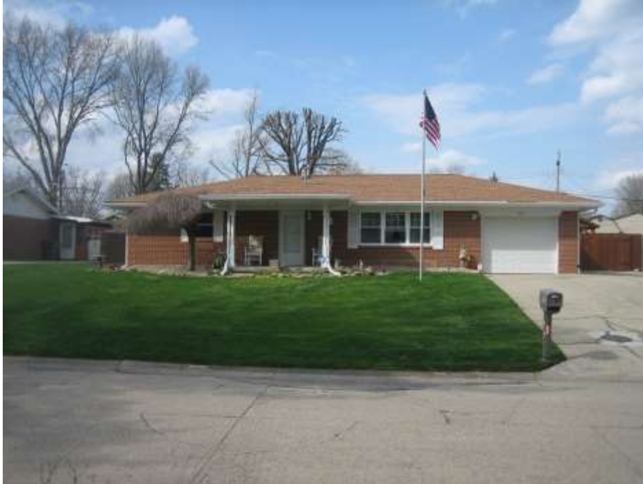
Subject property primary dwelling looking north.
