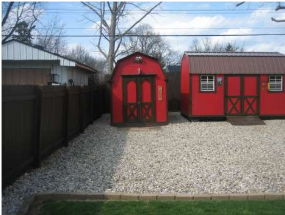
Subject accessory structure (left) encroaching into easement and west side setback, looking north.
