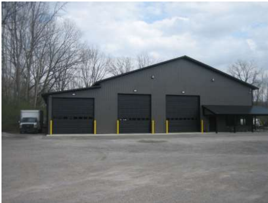
Subject site, existing office and storage building on site, looking east
