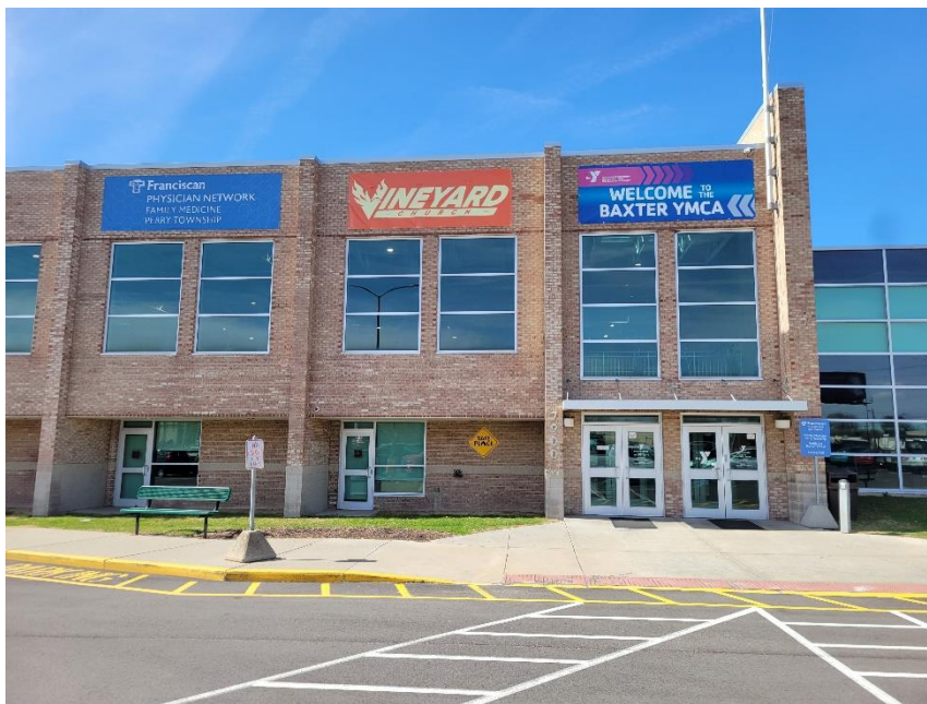
Photo 2: Primary YMCA Entry Viewed from East
