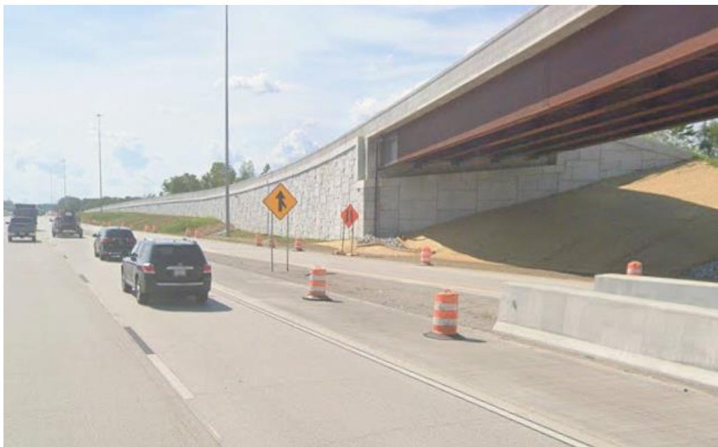
Photo 8: Same Location as Photo 5 but from August 2025 instead of July 2021
