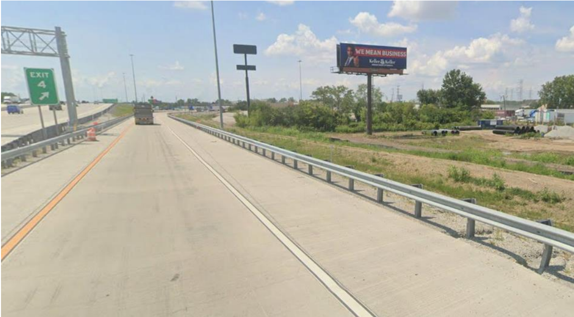
Photo 5: Existing Billboard on Western Portion of Subject Site (August 2025)
