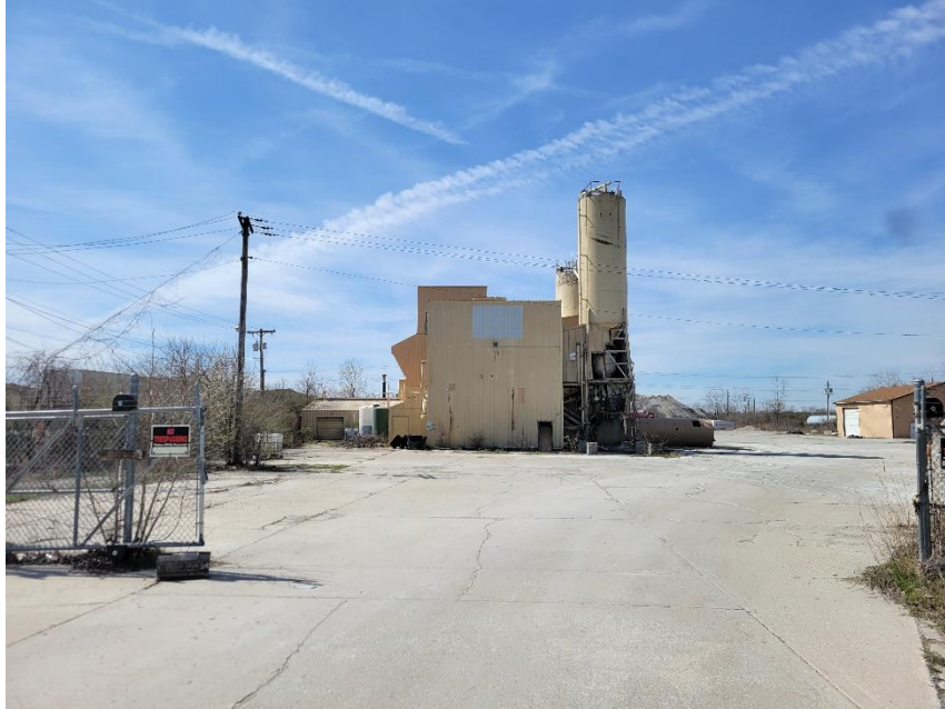
Photo 1: Subject Building Viewed from East
