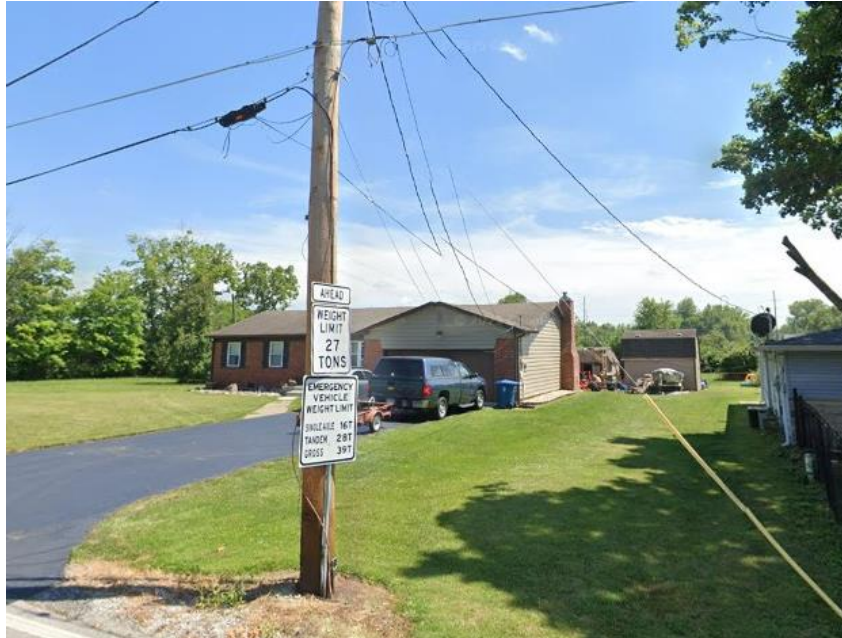
Photo 1: Subject Site Viewed from North (July 2024)
