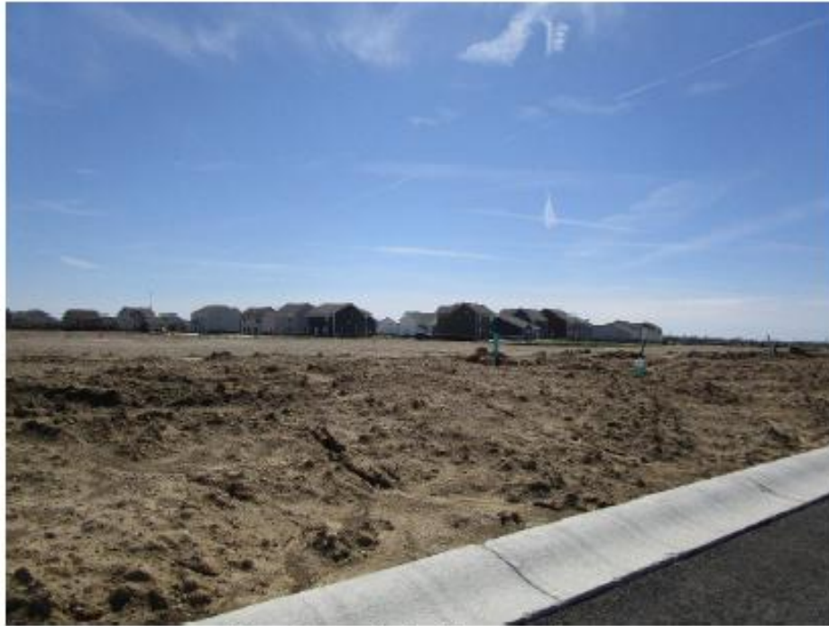
View from site looking southeast
