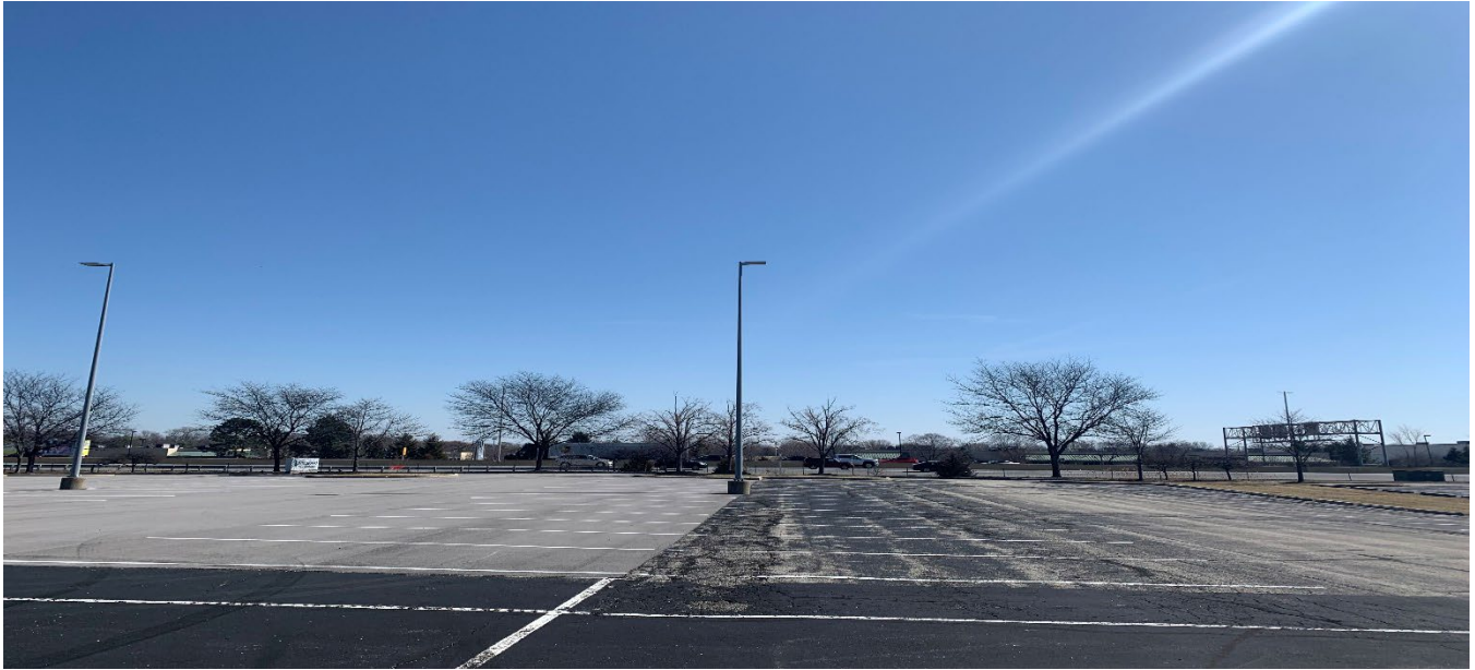
Photo of the parking area on site.
