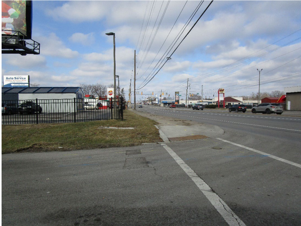
View looking north along North Keystone Avenue
