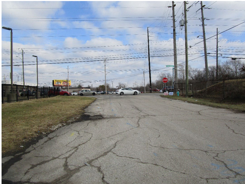
View looking east along Clay Street towards North Keystone Avenue
