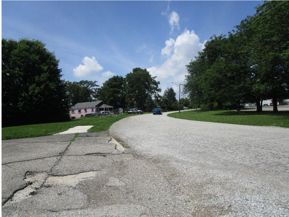
View looking north along South Ewing Street
