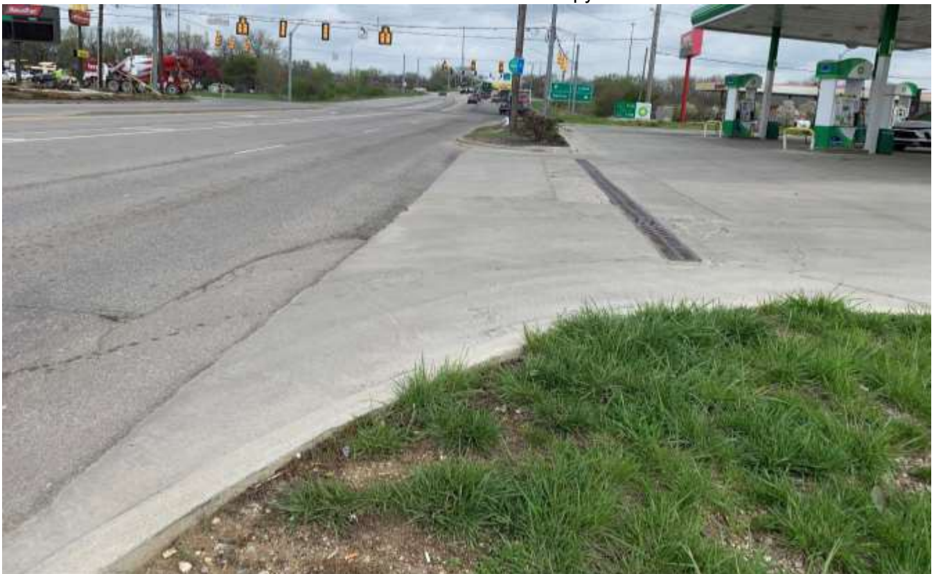
Photo of the street frontage along Holt Road looking north.
