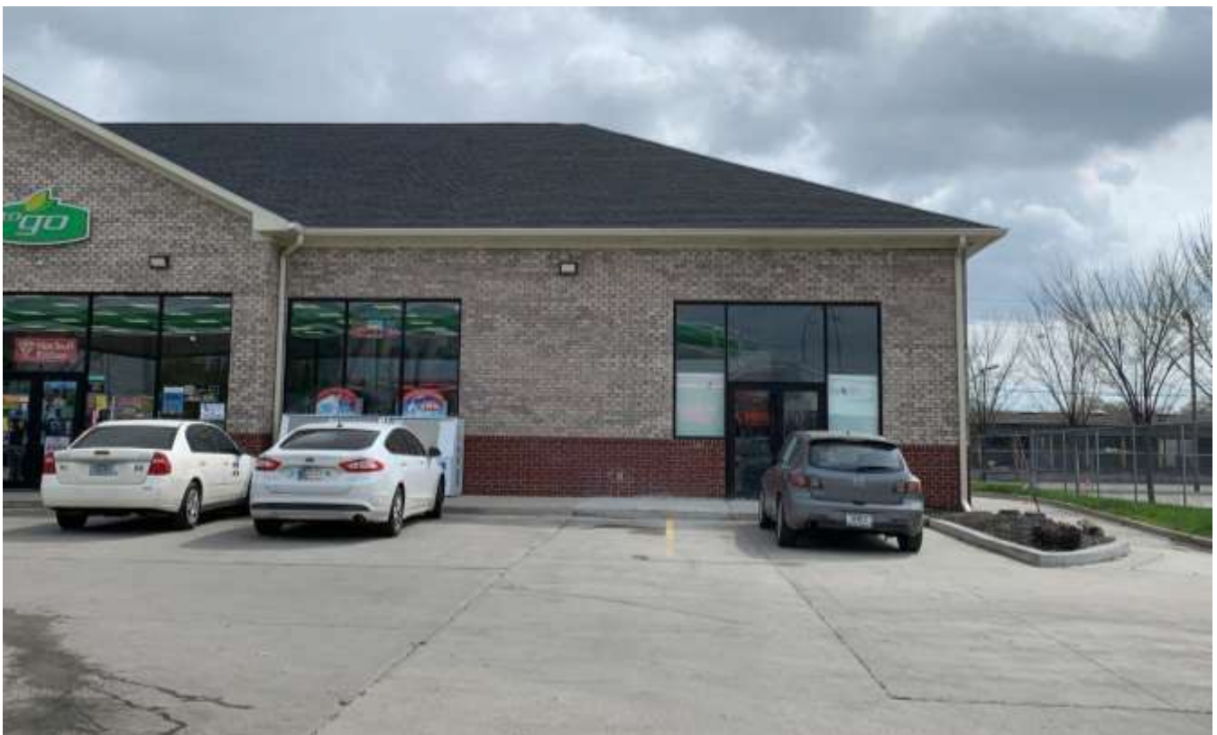
Photo of one of the empty tenant spaces.
