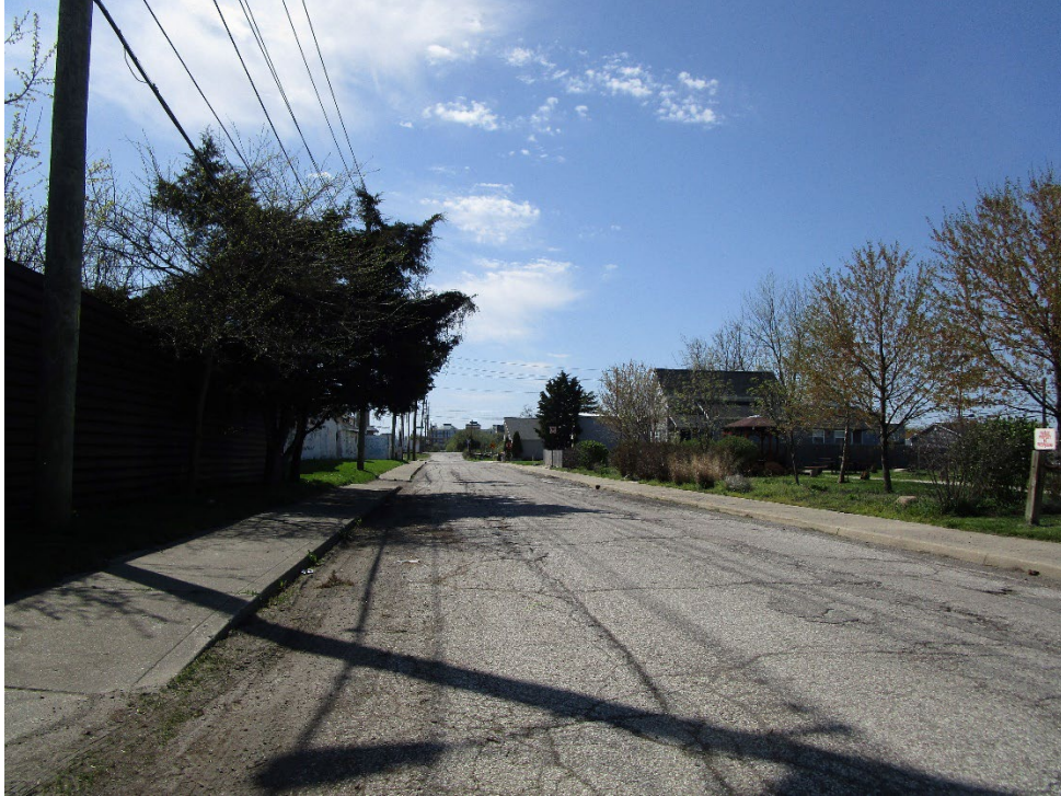
View looking west along Bates Street
