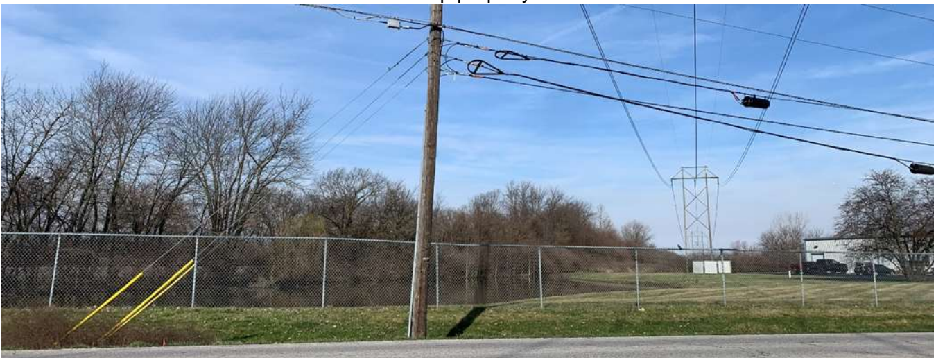
Photo of the machine shop property southeast of the site and southern transmission tower easement.
