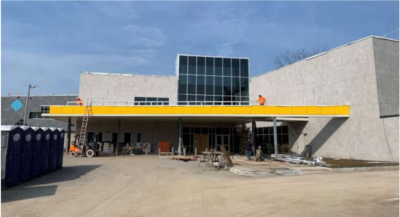
Photo of the canopy and proposed sign location looking west.
