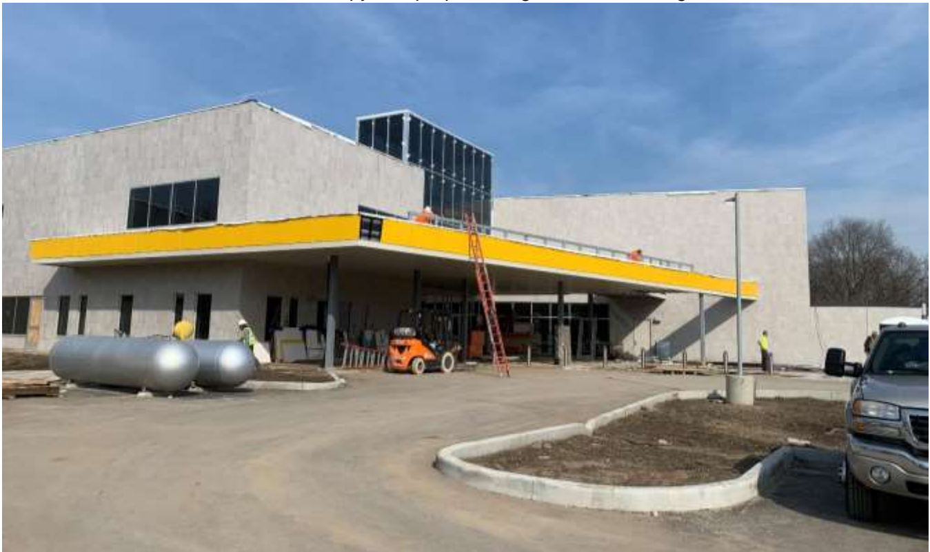
Photo of the canopy and proposed sign location looking north.
