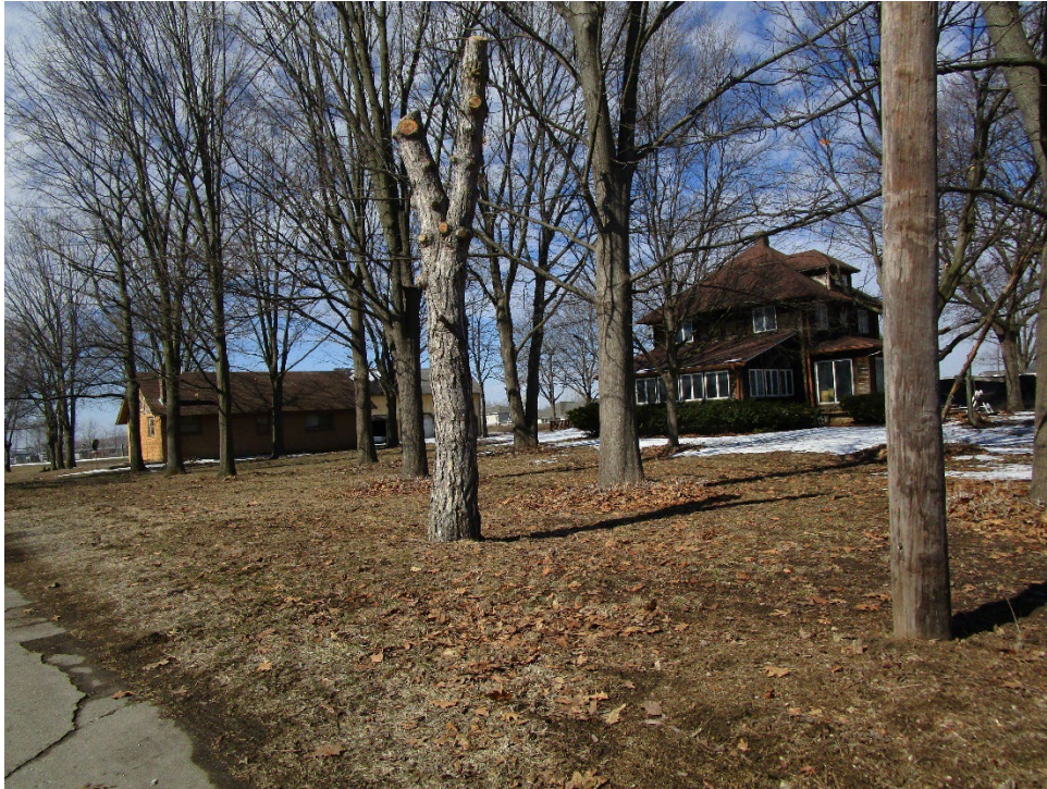
View of site looking northwest
