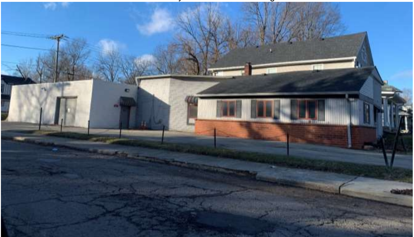
Photo of the building east of the site that the parking lot would be associated with.
