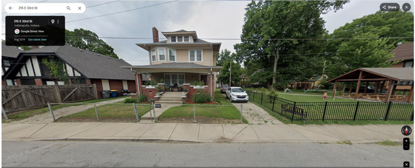
Photo 2: Google Image of subject site in 2019
