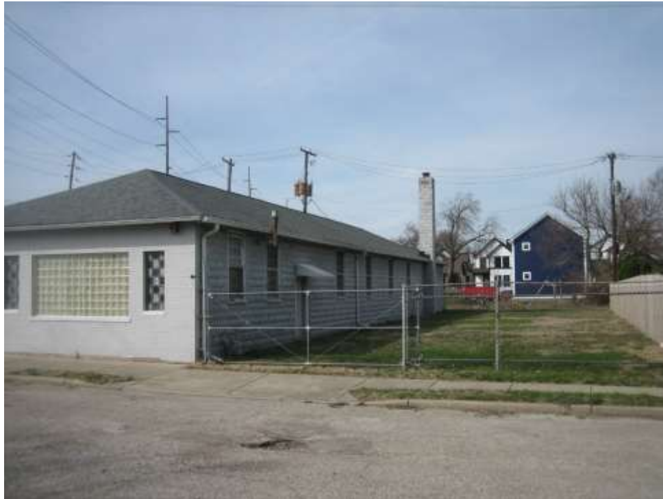
Adjancet Industrial use to the north.
