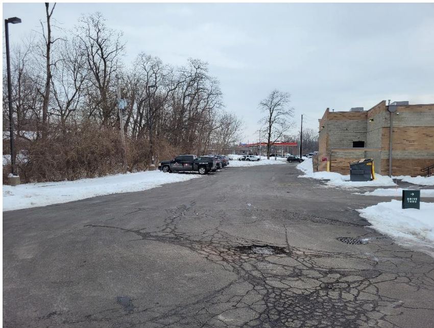
Photo 4: Existing Parking Area to South of Structure
