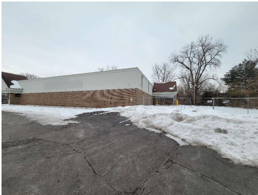
Photo 2: Current Structure Viewed from Southeast
