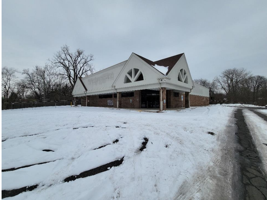
Photo 1: Current Structure Viewed from Southwest
