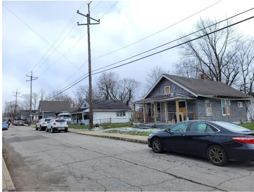
Photo 9: Adjacent Property to Southeast
