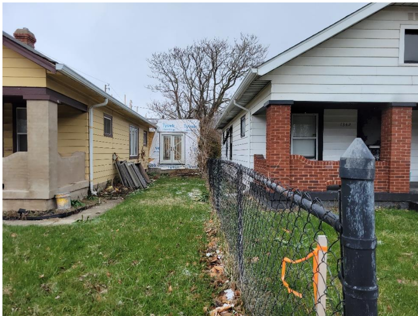
Photo 6: Addition Viewed from Eastern Property Line
