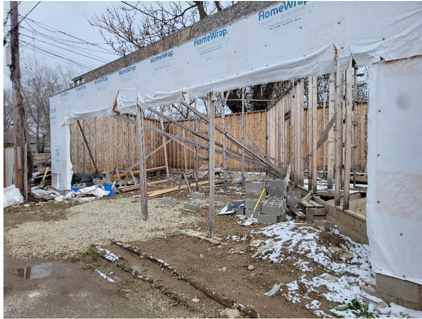
Photo 3: Subject Site Viewed from West
