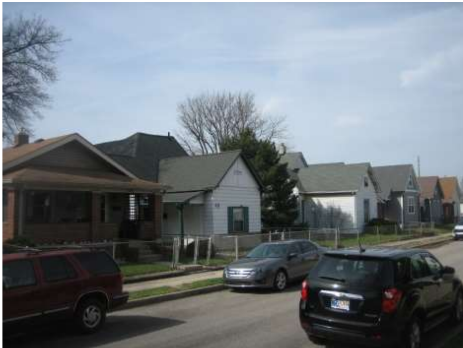
Adjacent dwellings to the northwest of site.
