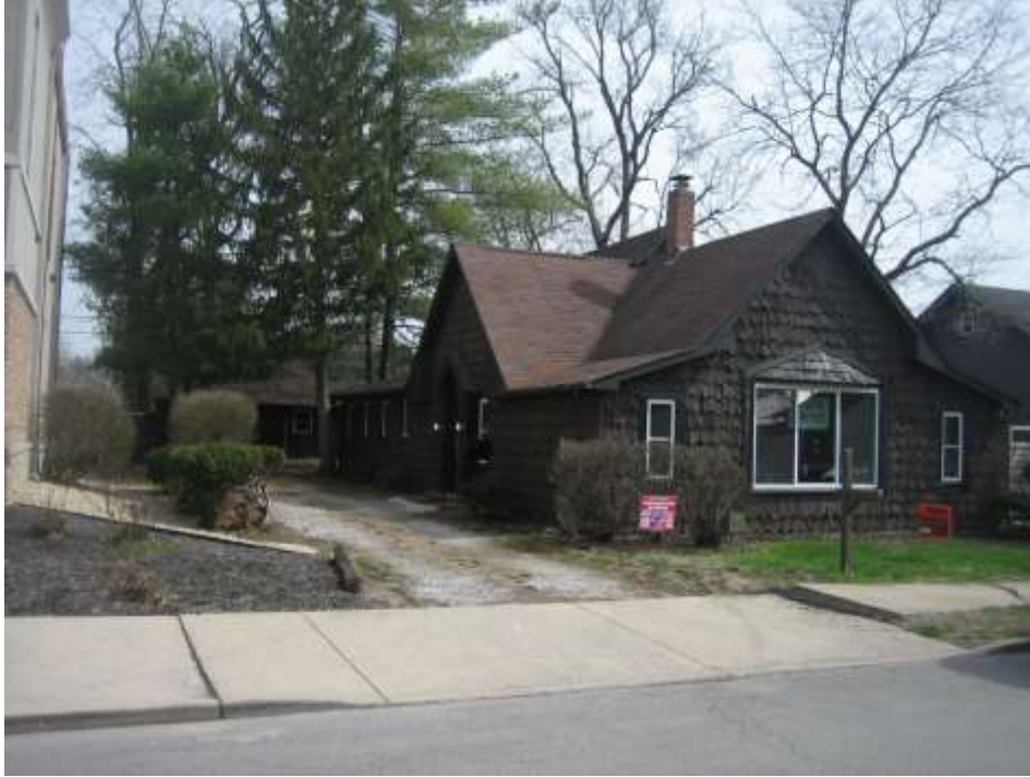
Subject site existing building, looking east.
