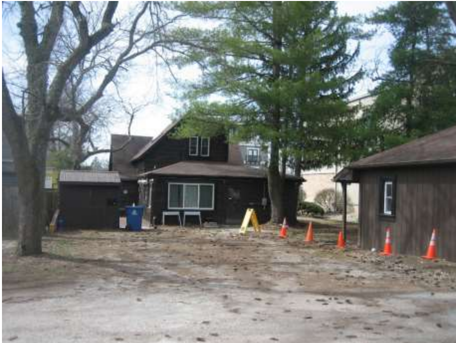
Subject site, rear of parcel looking west.
