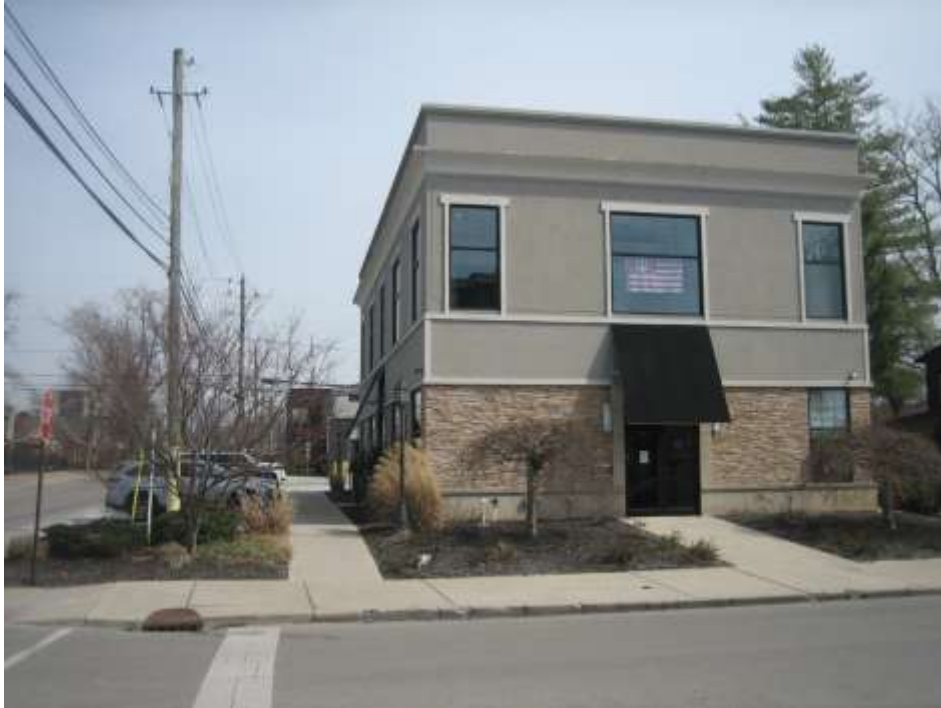
Adjacent commercial uses to the north, looking east
