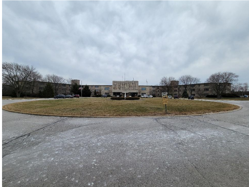
Photo 1: Subject Site Viewed from North
