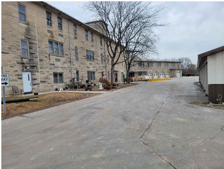
Photo 4: Current Building Viewed from West
