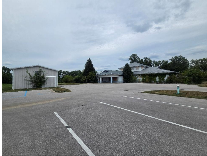
Photo 1: Existing Buildings Viewed from Southwest
