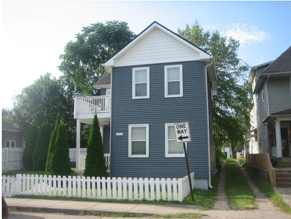
Photo of adjacent property to the east, looking south.
