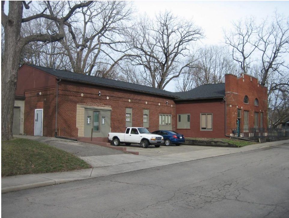
Photo of adjacent triplex dwelling to the north, looking northeast.
