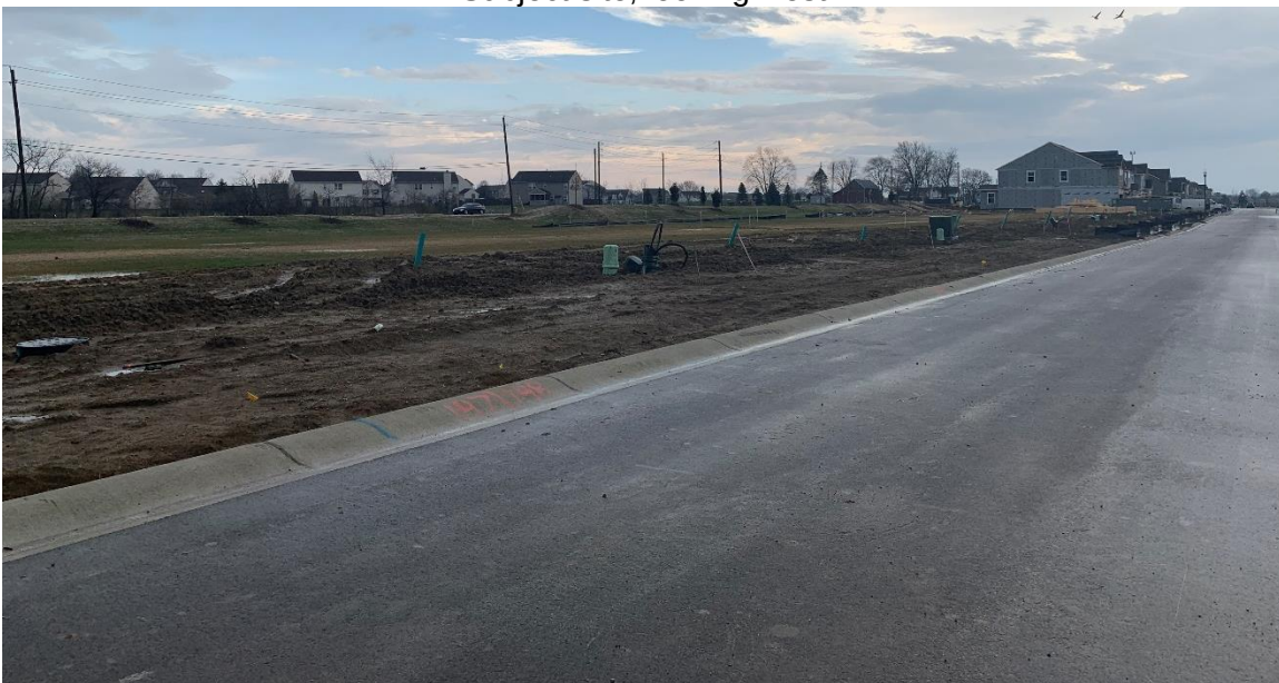
46 th Street frontage, looking east
