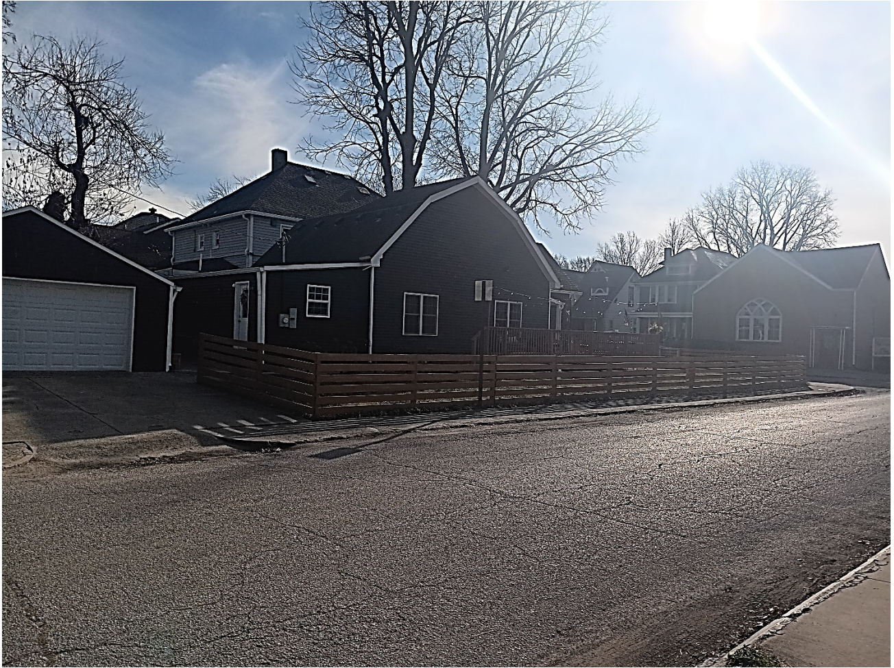
Exhibit 6: 1502 Pleasant Street looking at the home and fence from across Spruce Street.
