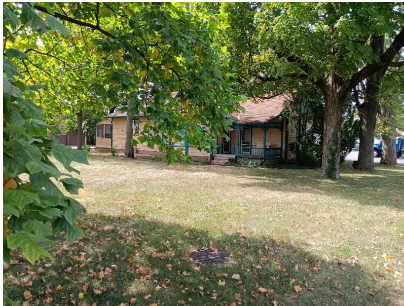
Exhibit 13: The dwelling to the west of the proposed contracting business.
