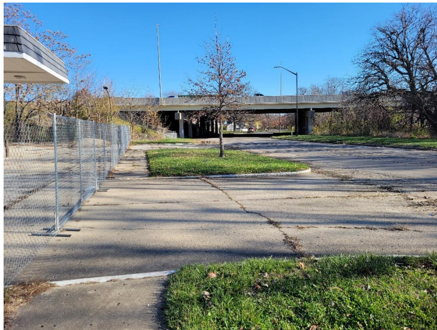
Photo 8: Existing Curb Cuts along Pleasant Run Pkwy NDR
