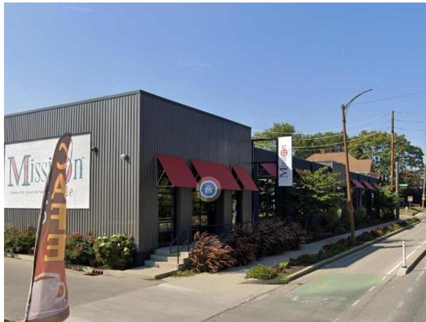
Photo 6: Adjacent Property & Bike Plane to the Northwest (September 2024)
