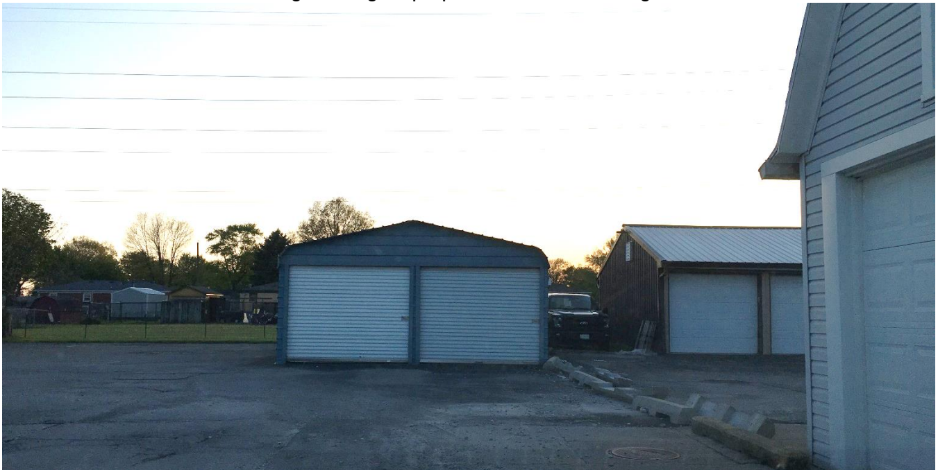
Existing building on proposed Lot One, looking west
