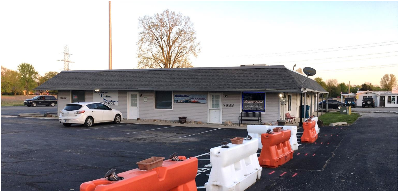
Existing building on proposed Lot Two, looking south
