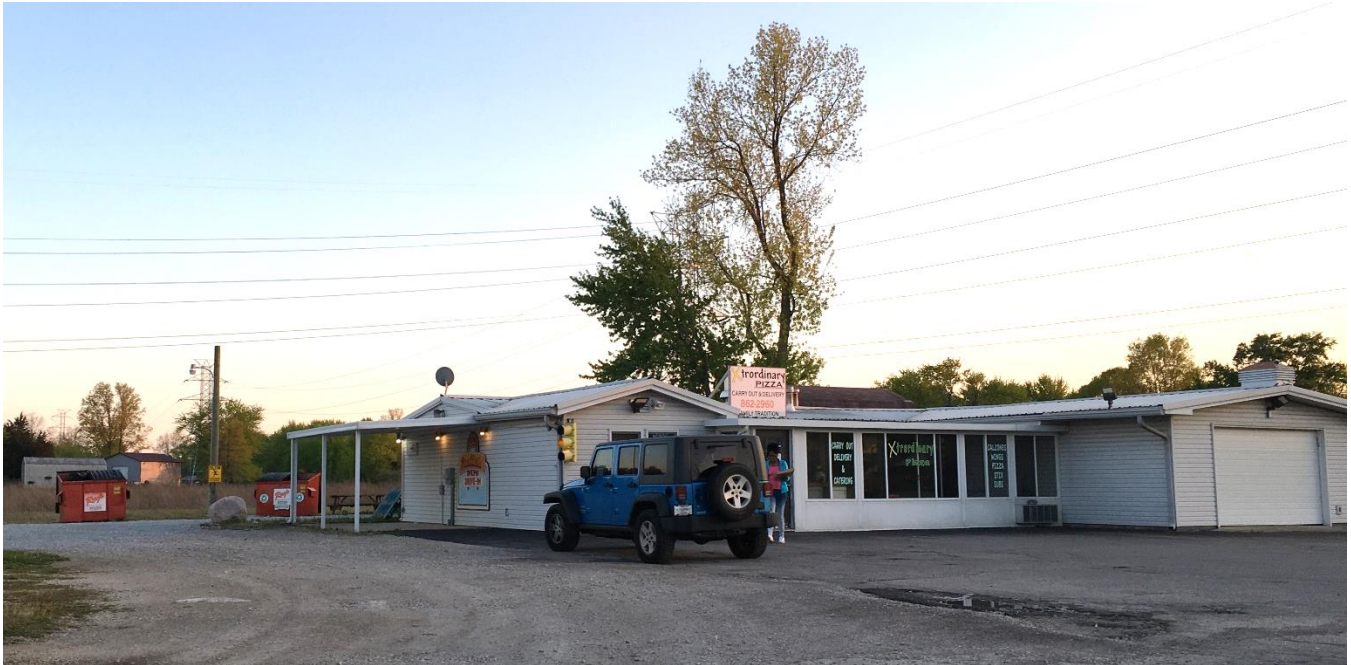
Existing building on proposed Lot One, looking south
