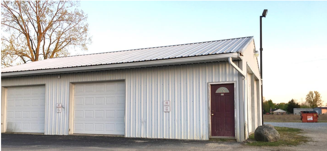
Existing building towards the rear on Proposed Lot Two, looking south
