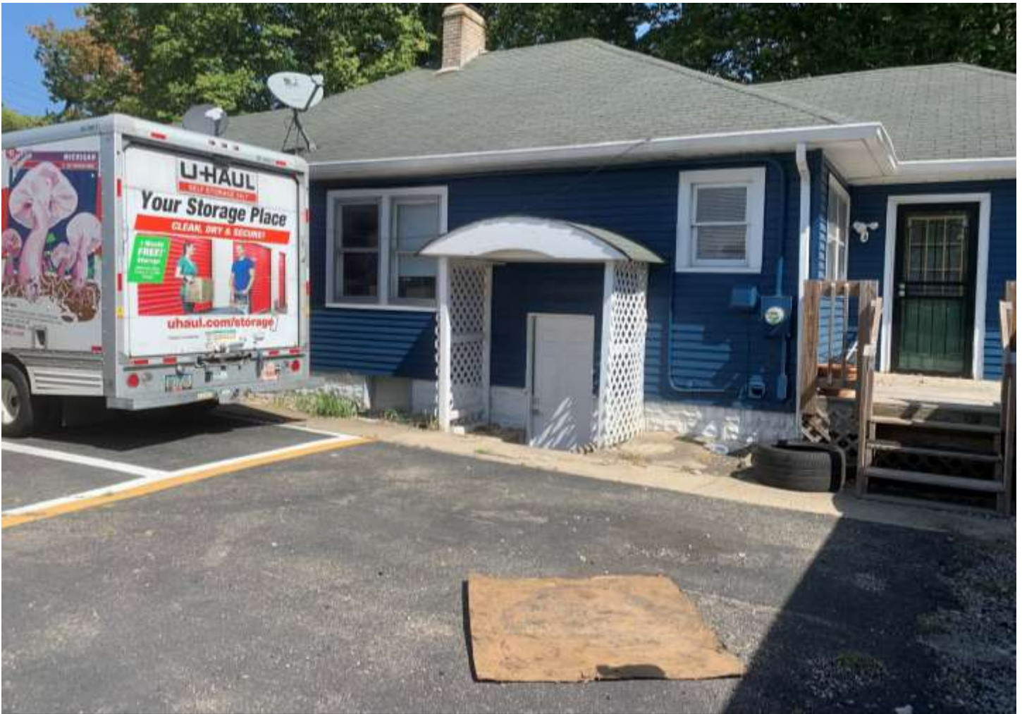
Photo of the western office façade.
