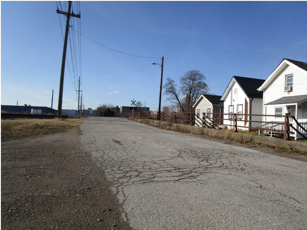
View looking west along Bates Street
