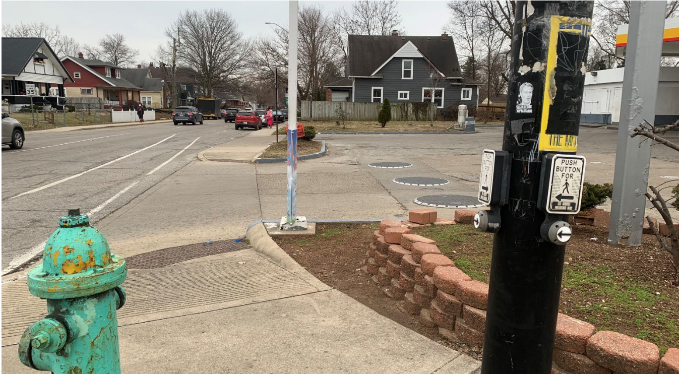
Street frontage along Capitol Avenue looking south.
