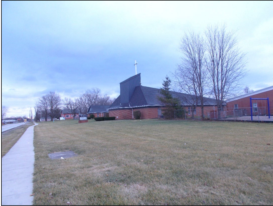
Looking east at the existing church building.
