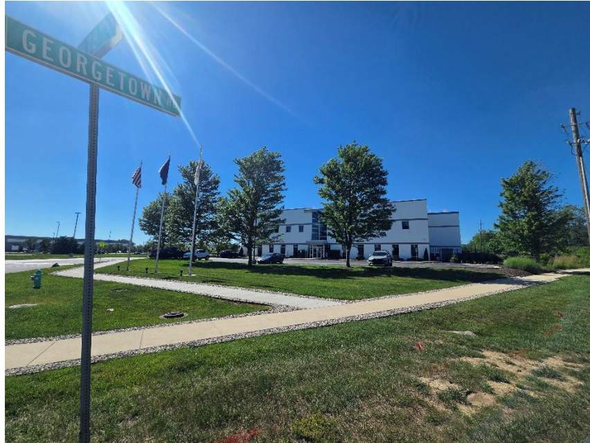
Photo 1: Northern Building Viewed from Southeast
