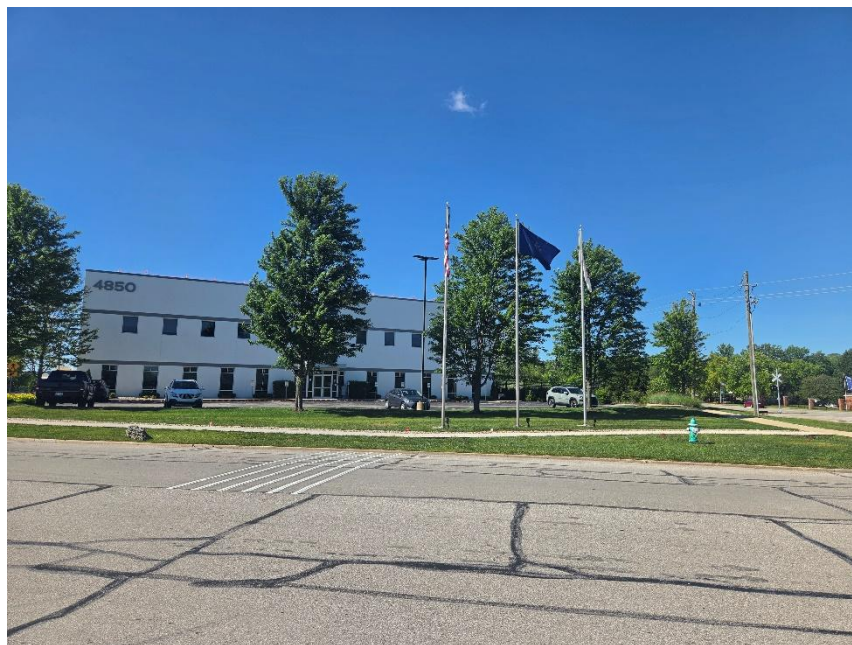
Photo 2: Northern Building Viewed from South
